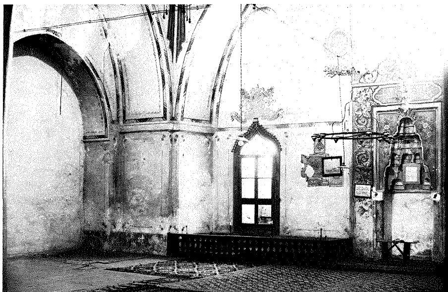
Fig. 11 — Jambol, Eski Cami, interior view
